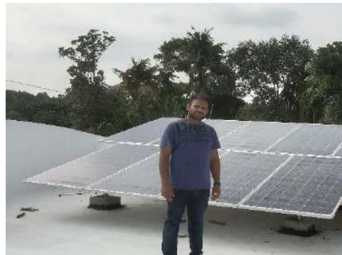
Jess Varghese 3 kWp
