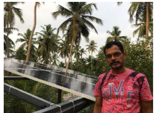
Ambujakshan A.K 3 kWp
